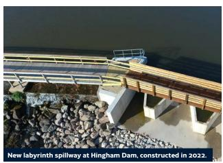
Hingham Dam impounds the Onion River in Sheboygan County, Wisconsin. According to a dam failure analysis (DFA) that we completed in 2019, Hingham Dam was incapable of passing the 100-year flood without overtopping. To be classified as a low-hazard dam in Wisconsin, among other criteria, the dam must pass the 100-year flood without overtopping its embankment.
